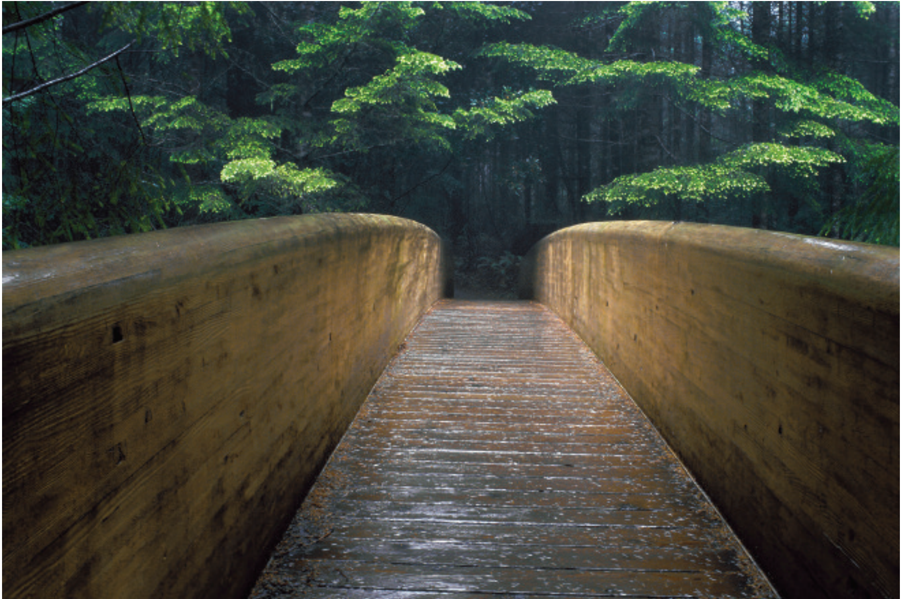
'BRIDGE TO SOMEWHERE' A walkway overpass in the Lady Bird Johnson Grove, Redwood National Park is enhanced by bright-diffused light during a wet winter day.
